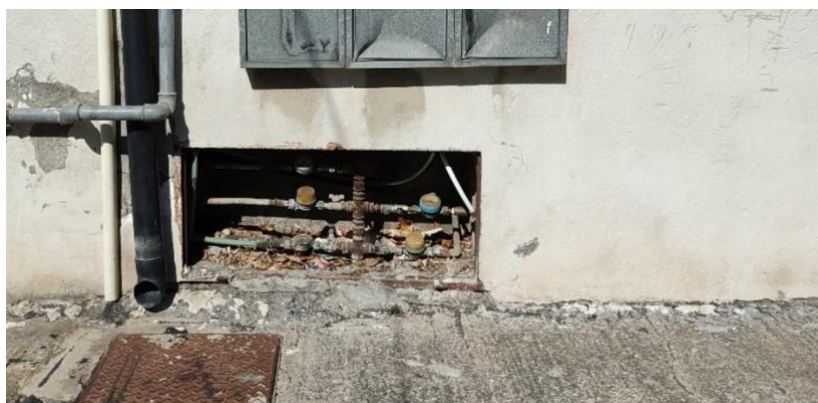
Figure 54: Water meters located at the east front of the building
