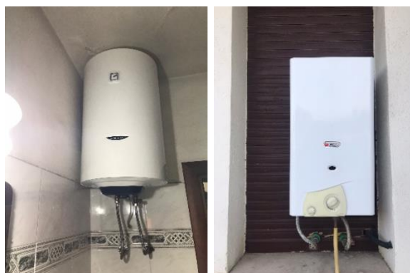
Figure 51: A typical electric boiler (on the left) and gas boiler (on the right) found in the pilot building for DHW production.
