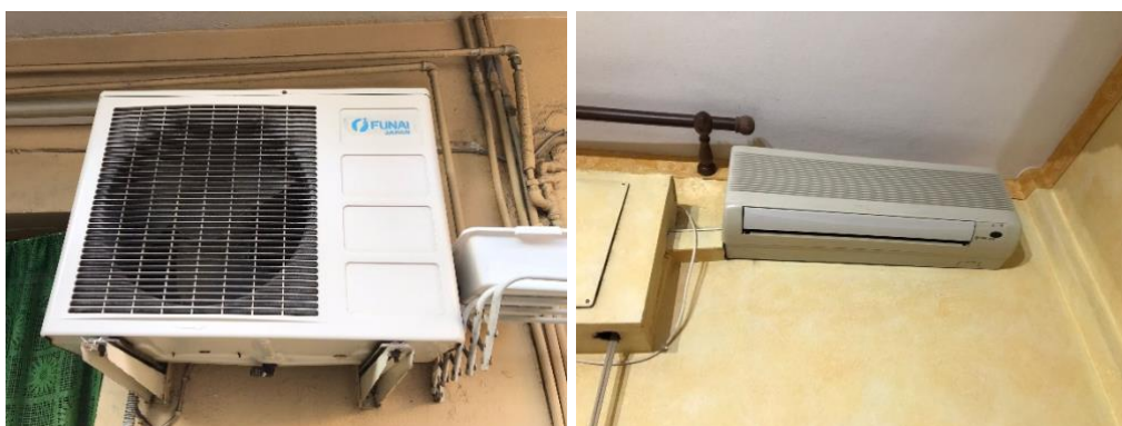
Figure 50: External (on the left) and internal (on the right) views of a split unit in flat 2L.
