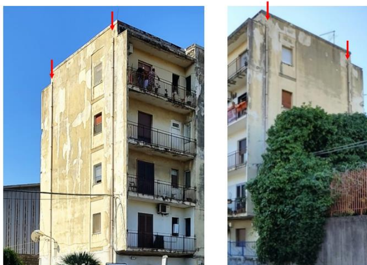
Figure 52: Downpipes placed on the east (left side) and west (right side) oriented facades of the pilot building
